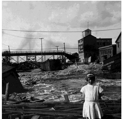
Stereogram picture shows one view of widespread damage from 1912 Flood.
